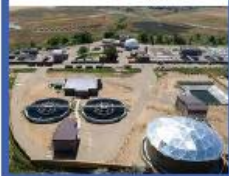
Lafayette Water Reclamation Plant
