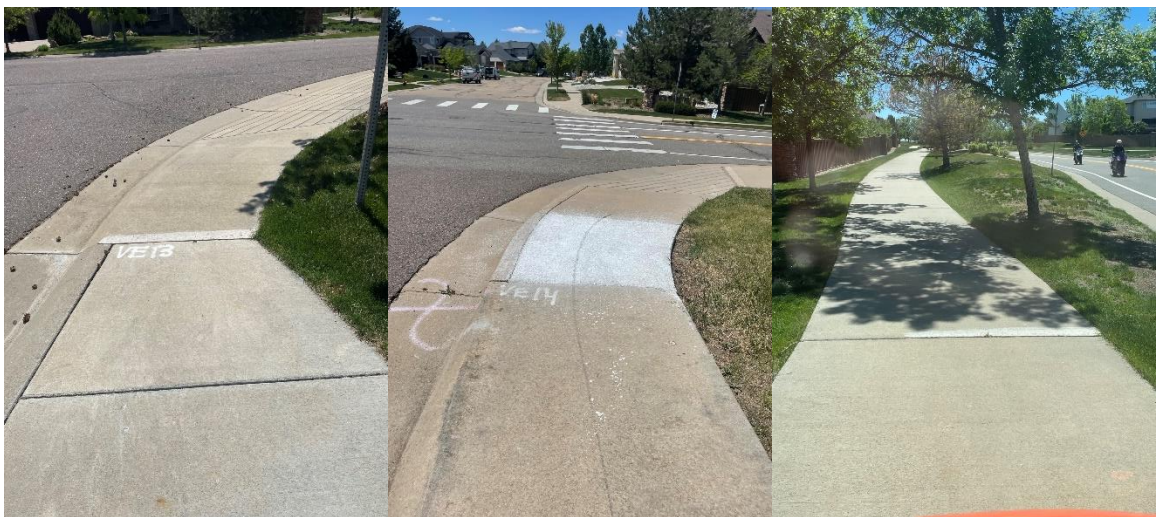
VE13, VE14, VE15 COMPLETED
