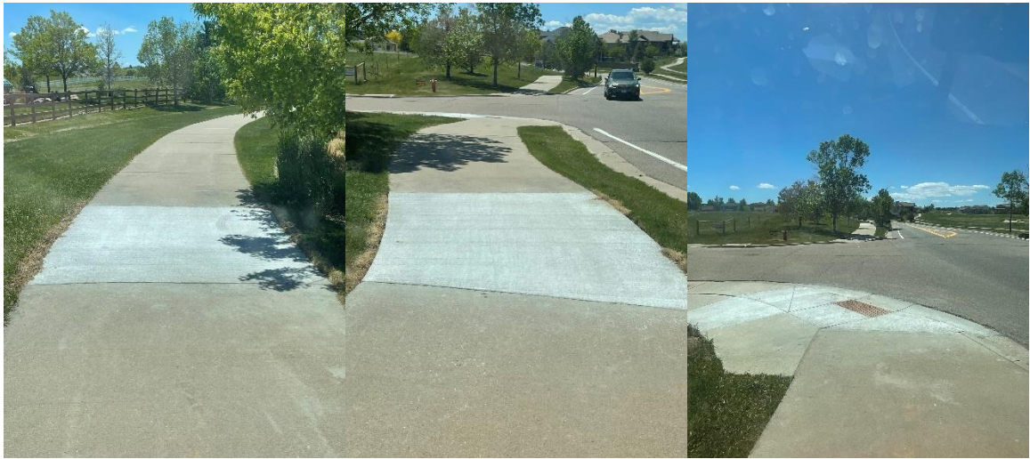
VE5, VE6, VE7, VE8, AND VE9 COMPLETED
